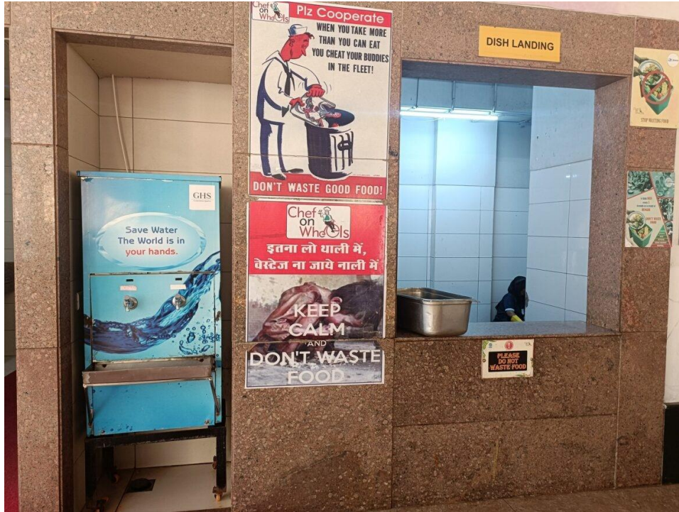
Picture 3: Water coolers installed in MUJ Hostel
